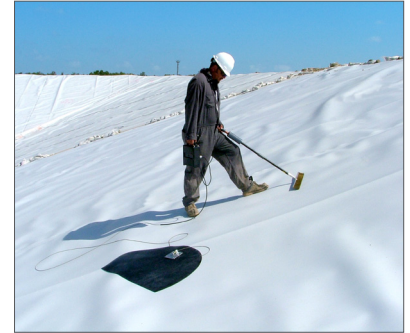
GSE Leak Location spark testing
