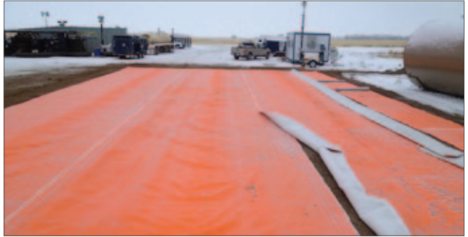
[ContainMat Installation]
