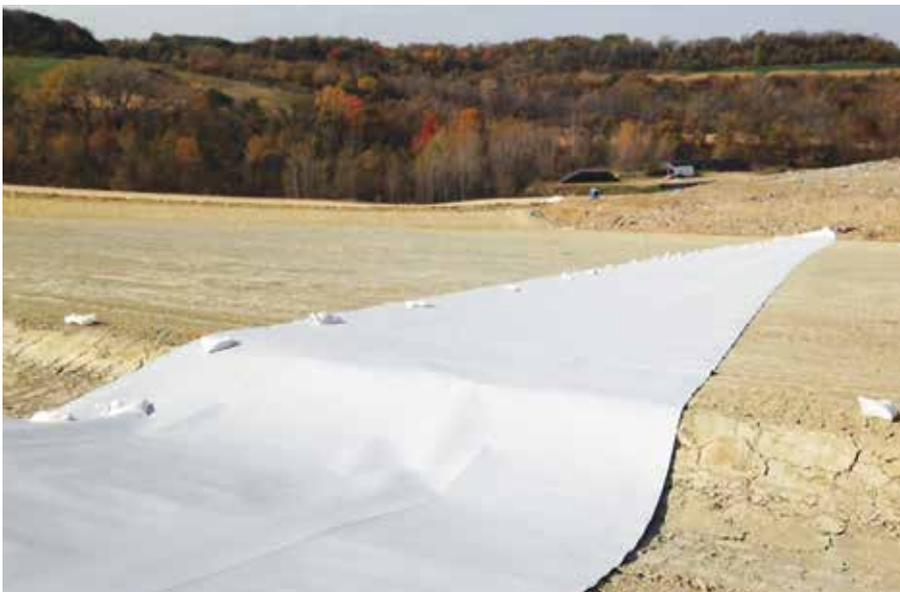
**PHOTO 5** White-surfaced HDPE geomembrane installed over compacted clay liner. Photo: AECOM
