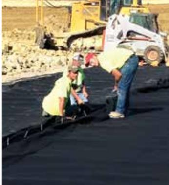
**PHOTO 2** Geonet overlapping and joined with cable ties. Photo: GSE
