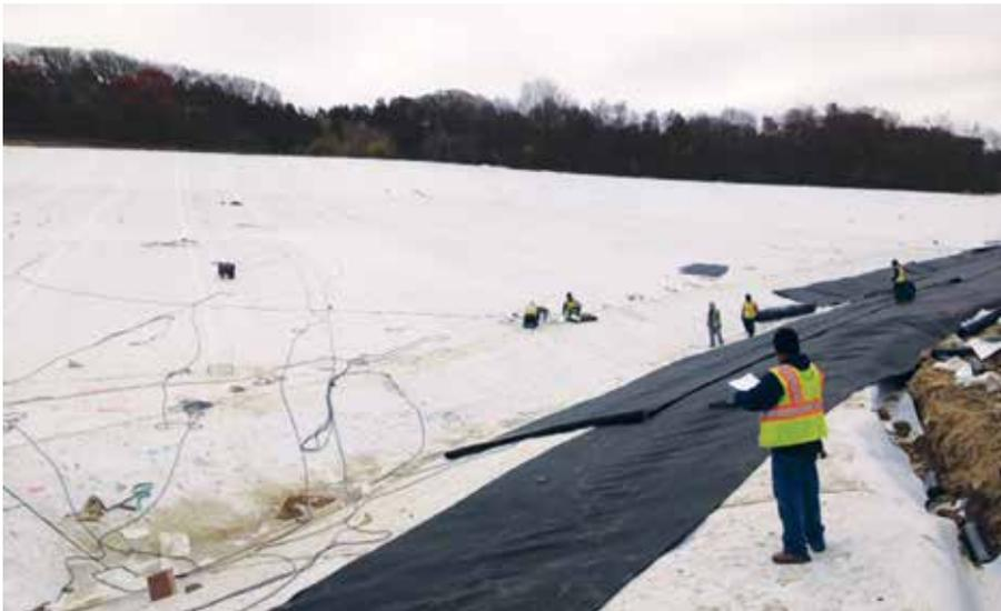
**PHOTO 4** White-surfaced HDPE geomembrane slope installation. Photo: AECOM
