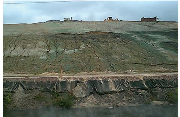
**Photo 1.** Slumps and erosion rill on a 2H:1V slope of a paper mill sludge landfill. From Richardson et al. (2004).
