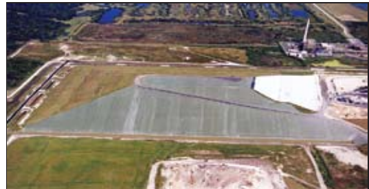
Completed 20 acre EGCS for a MSW landfill cover.
